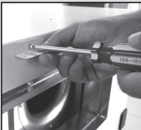
Figure 2: Bracket "A" Installed
